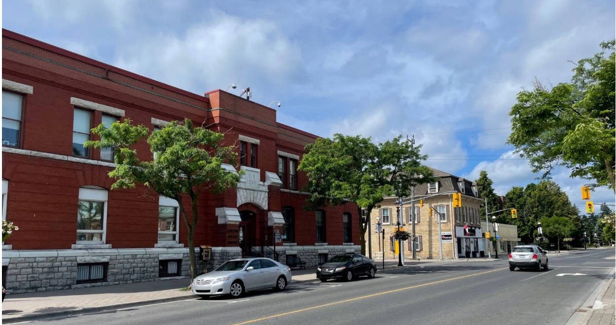
Fig. 4.1.1.1 – Existing Building at 107 King Street West
