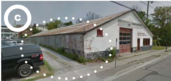
LOOKING EAST (QUEEN ST)
