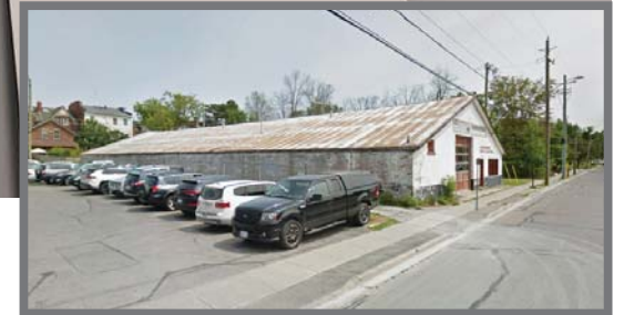
EXISTING 3M WIDE LANEWAY ACCESS
